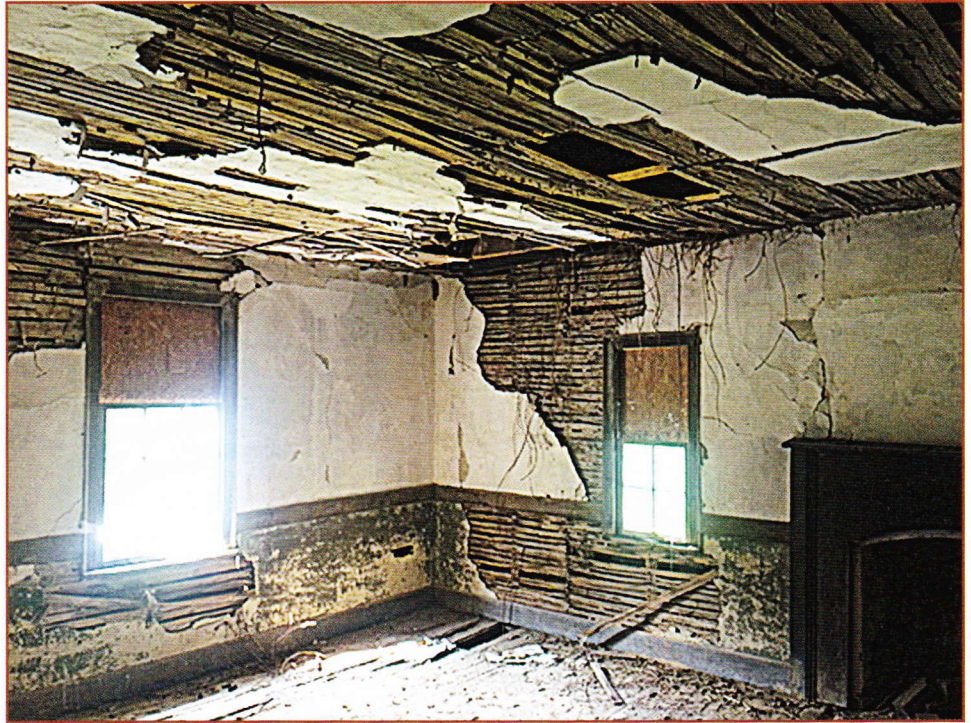
The current state of the inside of the Edward Dromgoole House. This is the original plaster. King said he would like to reuse as much of the lath (thin, flat strips of wood providing a foundation for the plaster) as he can.
